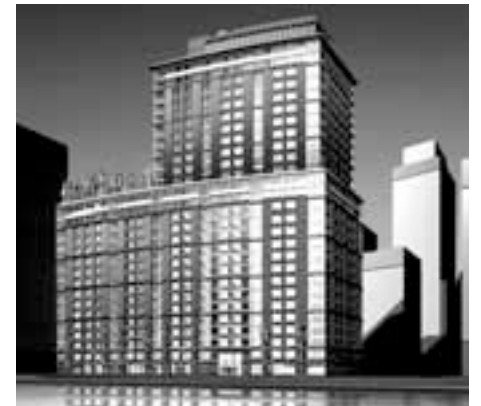
Battery Park City
