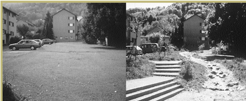
Before and after views of a Swiss daylighting project.
