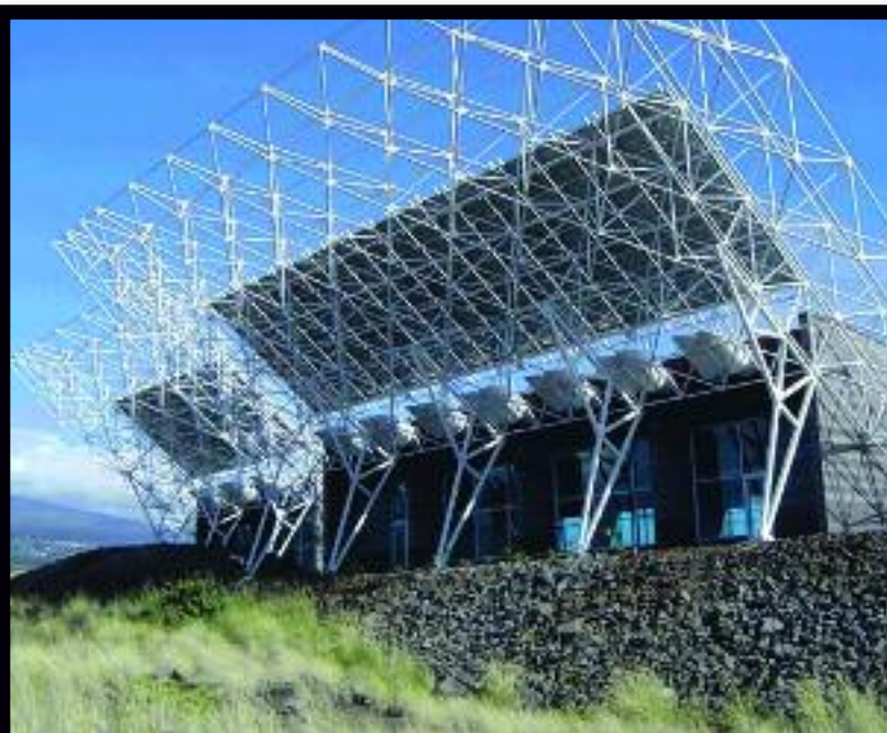
The Hawaii Gateway Energy Center (NELHA) visitor complex. The building is cooled by pumped seawater, and all the necessary energy is provided by the PV array.
