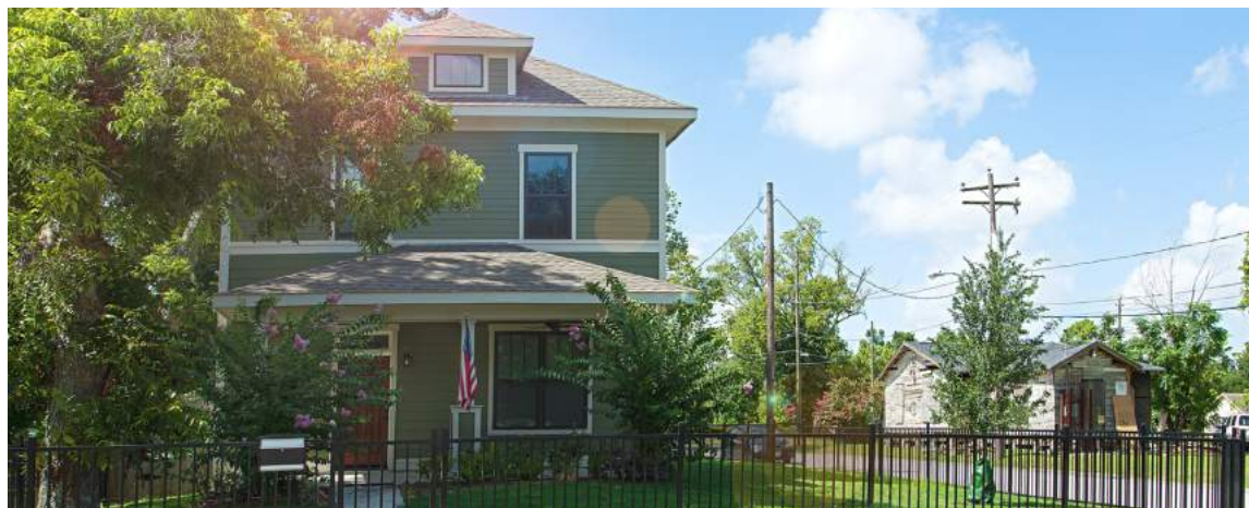
A recently completed net-zero home shows what the future will look like for the run-down shack in the background, one of the next the HOUZE team is tackling.
